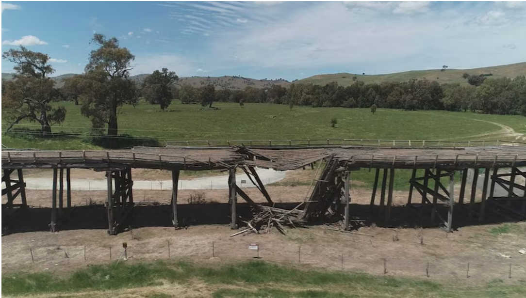
Gundagai Prince Alfred timber bridge prior to demolition. (ABC Riverina: Simon Wallace)
